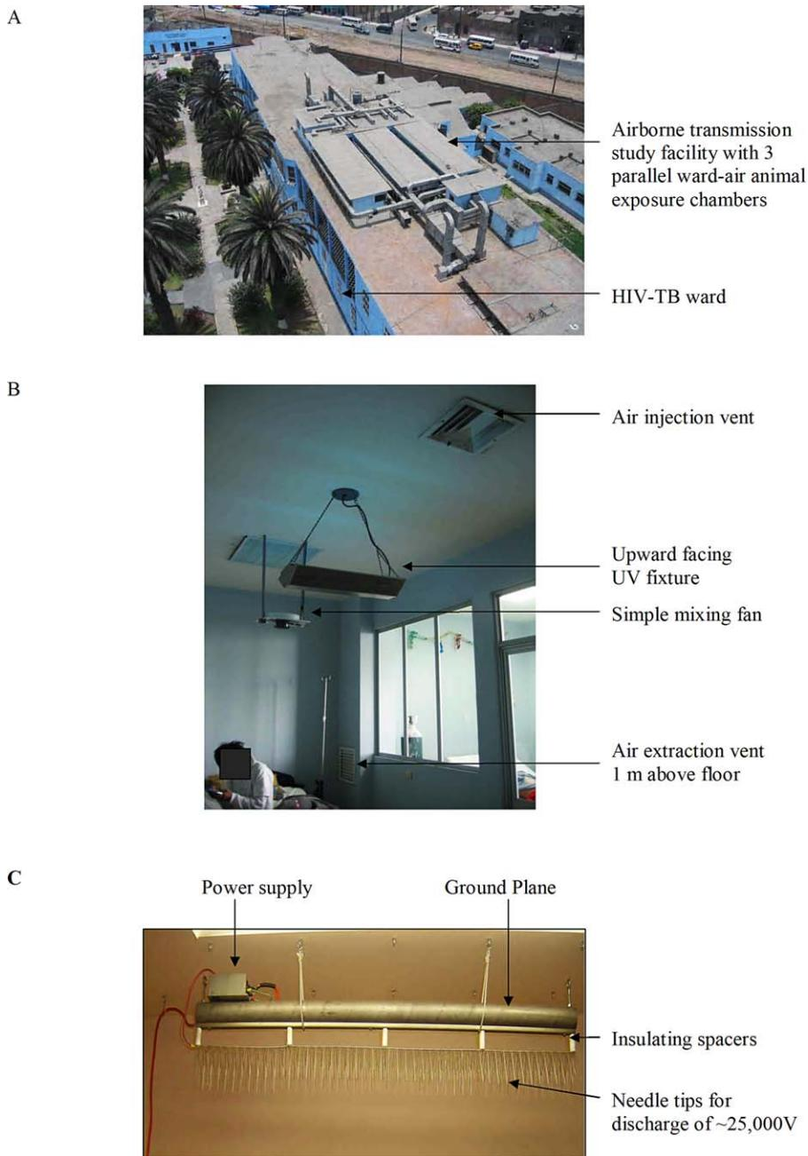
**Figure 1.** Bird's Eye View of Guinea Pig Air Sampling Facility on Roof of HIV-TB Ward; Photograph of HIV-TB Isolation Room Showing UV Light Fixture, Mixing Fan, and Ventilation System; and Photograph of Large-Scale ESCS Ionizer
